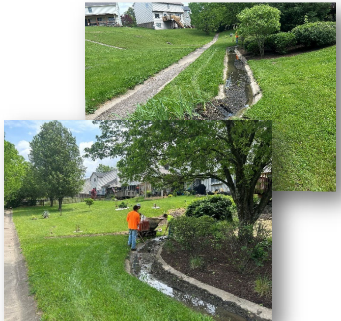
Cleaning Concrete Stormwater Flumes
