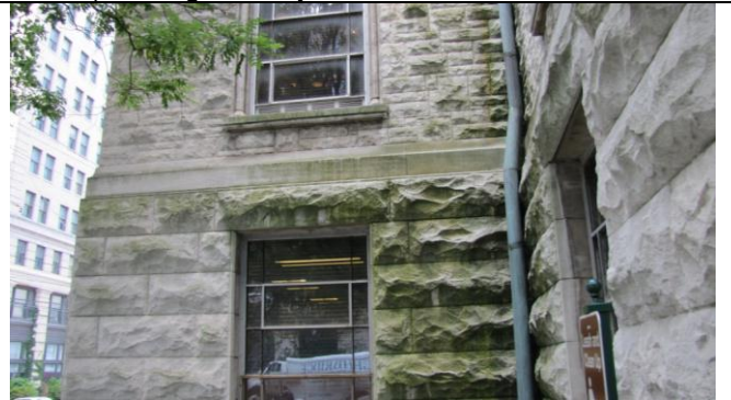
Photograph #28: First floor Public Safety Room below Photograph #27
