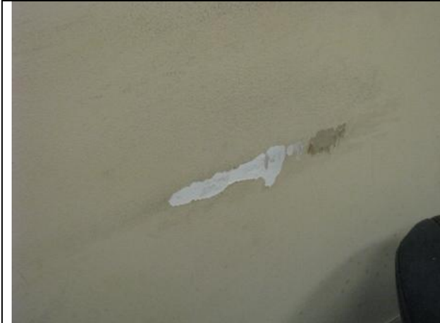
Photograph #9: Paint sample location for 2 nd floor wall (P-8).
