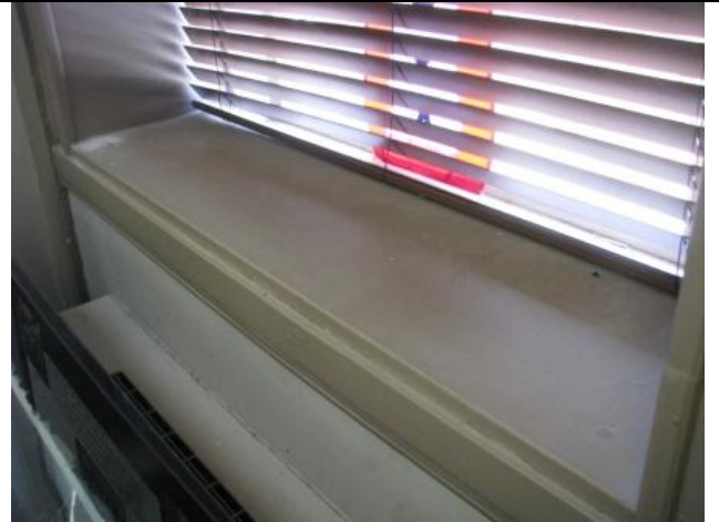
Photograph #38: Wipe sample location from 2 nd floor window sill (W-25).
