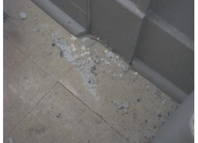
Photograph #34: 2 nd floor wipe sample location from floor (W-20).
