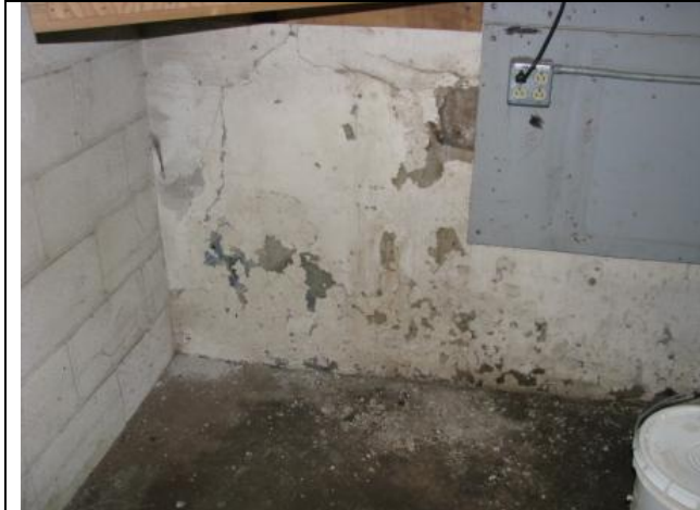
Photograph #13: Paint sample location for basement wall (P-12).
