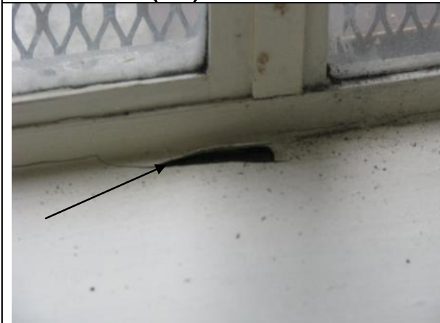
Photograph #11: Paint sample location for 1 st floor window sill (P-10).
