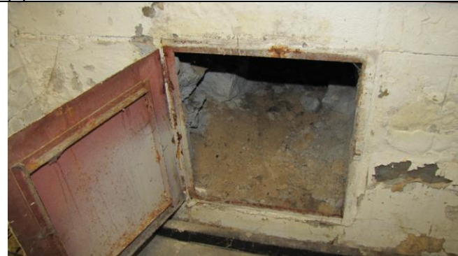
Photograph #7: Access crawlspace at basement hallway near stairway
