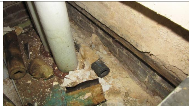
Photograph #5: Construction of exterior wall inside pipe chase
