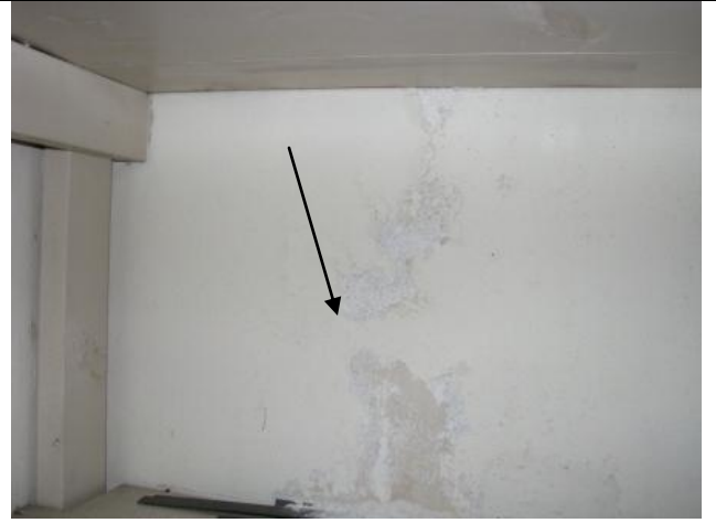
Photograph #6: Paint sample location for 4 th floor wall (P-5).
