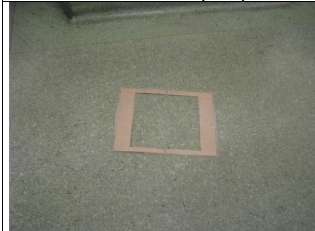
Photograph #27: 3 rd floor wipe sample location from hallway floor (W-13).
