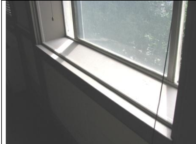
Photograph #25: Wipe sample location from 3 rd floor window sill (W-11).
