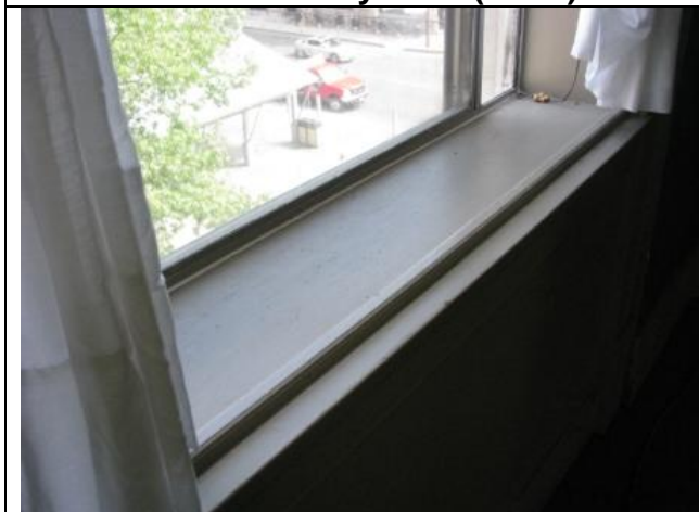
Photograph #29: Wipe sample location from 3 rd floor window sill (W-15).
