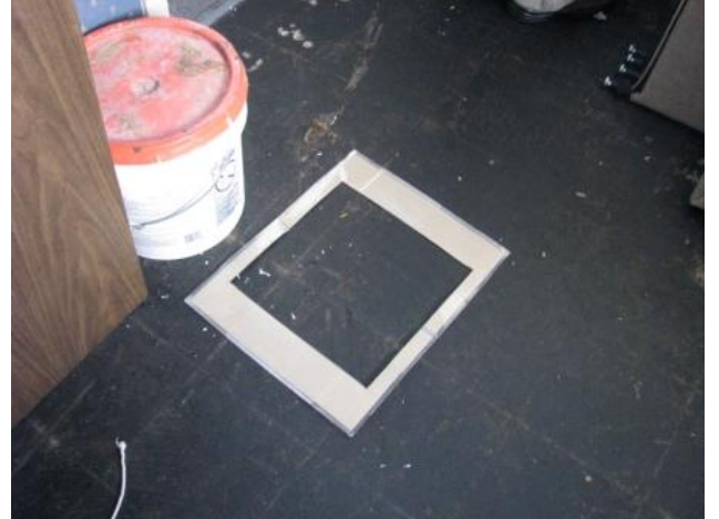
Photograph #32: 3rd floor wipe sample location from floor (W-18).
