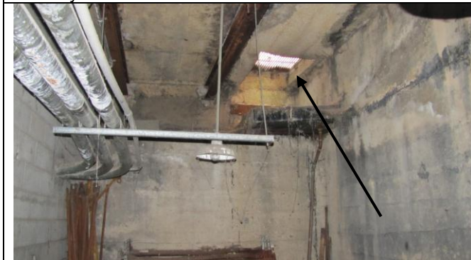
Photograph #9: Basement open grate near building
