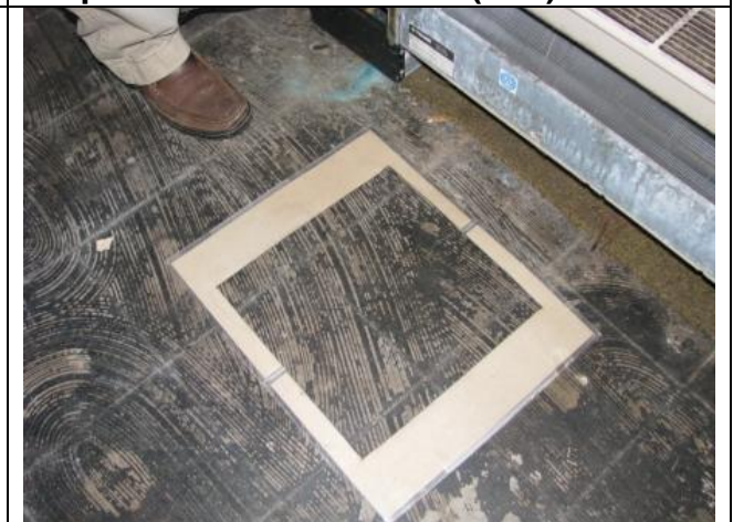
Photograph #18: 4 th floor wipe sample location for floor (W-4).
