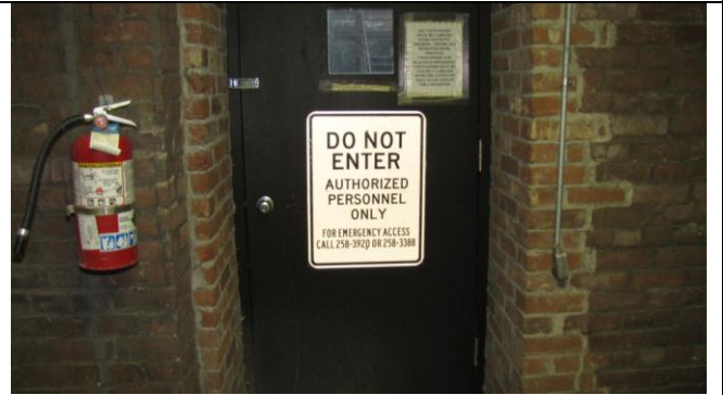
Photograph #14: Penthouse entrance
