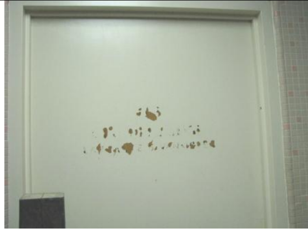
Photograph #5: Paint sample location for 4 th floor door (P-4).
