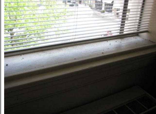
Photograph #31: Wipe sample location from 3rd floor window sill (W-17).
