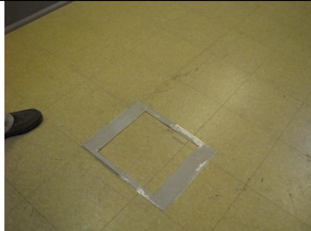
Photograph #39: 2 nd floor wipe sample location from floor (W-26).
