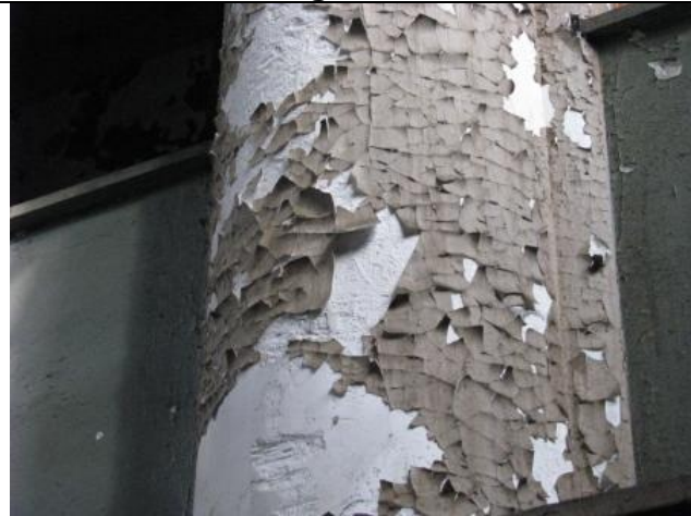
Photograph #3: Paint sample location for penthouse column (P-2).
