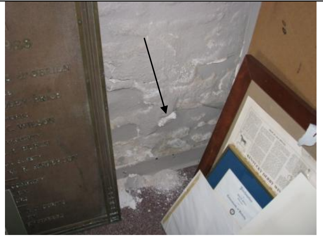
Photograph #4: Paint sample location for 4 th floor wall (P-3).
