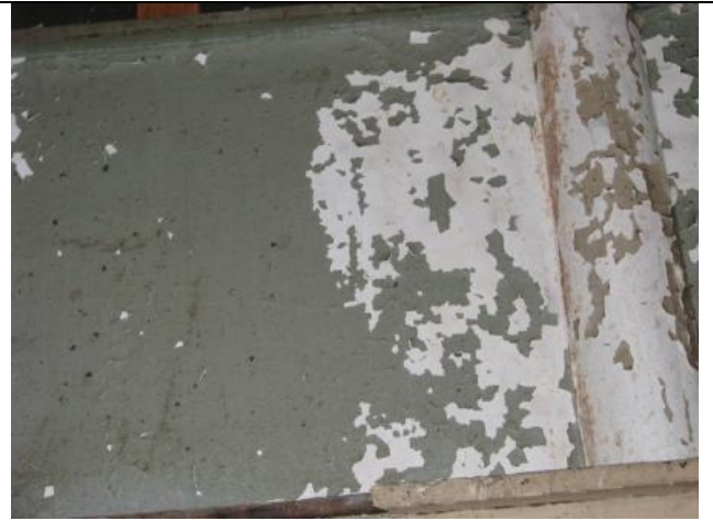
Photograph #2: Paint sample location for Penthouse wall (P-1).
