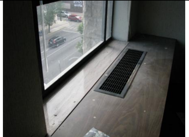
Photograph #20: Wipe sample location from 4 th floor window sill (W-6).
