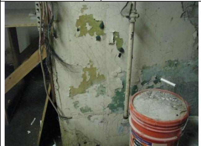
Photograph #12: Paint sample location for basement wall (P-11).
