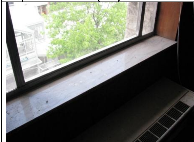
Photograph #17: Wipe sample location for 4 th floor window sill (W-3).
