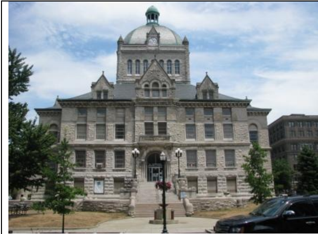
Photograph #1: Front view of 215 West Main Street, Lexington, KY.
