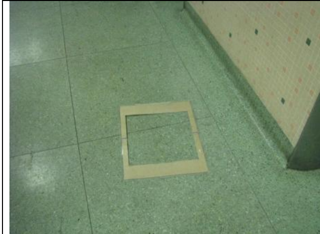
Photograph #19: 4 th floor wipe sample location from hallway floor (W-5).
