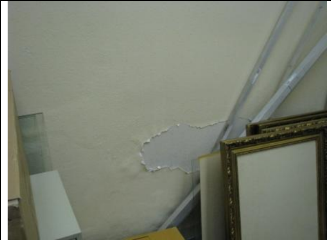
Photograph #10: Paint sample location for 1 st floor wall (P-9).
