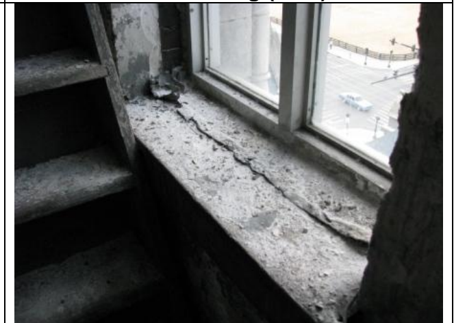
Photograph #16: Wipe sample location for penthouse window sill (W-2).
