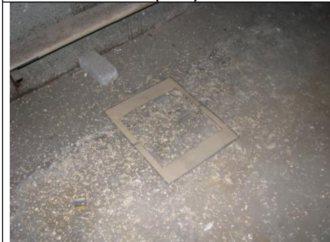
Photograph #15: Wipe sample location for penthouse floor (W-1).
