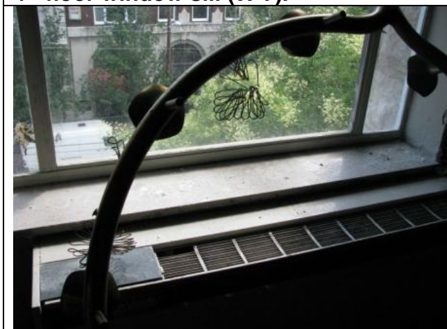
Photograph #23: Wipe sample location from 4 th floor window sill (W-9).
