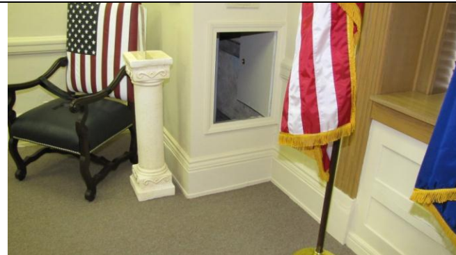
Photograph #3: Pipe chase in Fallen Heroes Memorial Room
