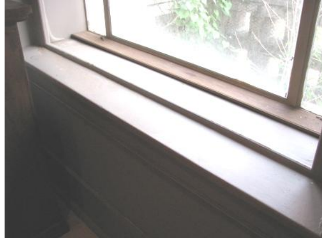
Photograph #33: Wipe sample location from 2 nd floor window sill (W-19).
