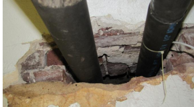
Photograph #15: Inner wall construction near corner in Fallen Heroes Room
