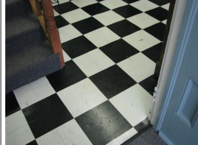
Photograph #43: 1 st floor wipe sample location from floor (W-30).
