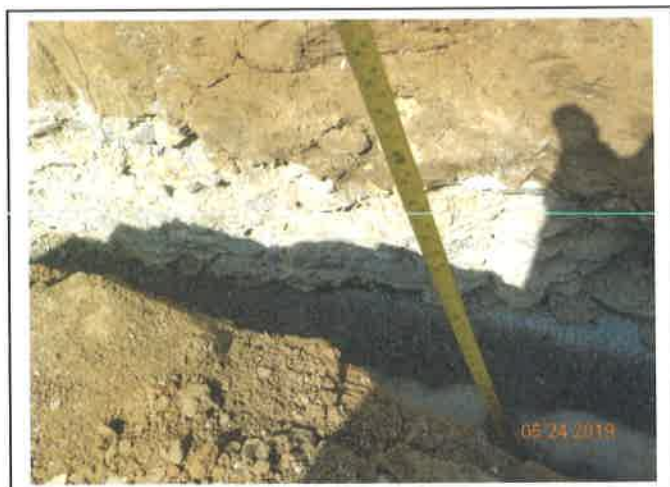
Photo #003 – Measuring depth (typical)
