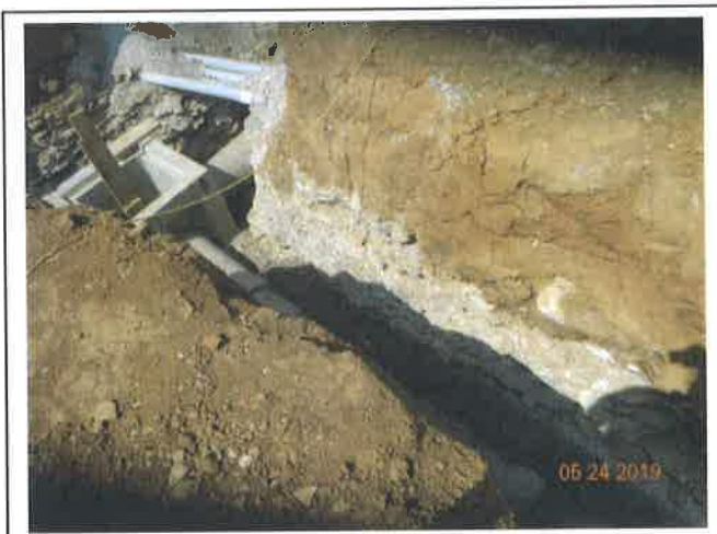
Photo #002 – CB2 to CB4 rock excavation
