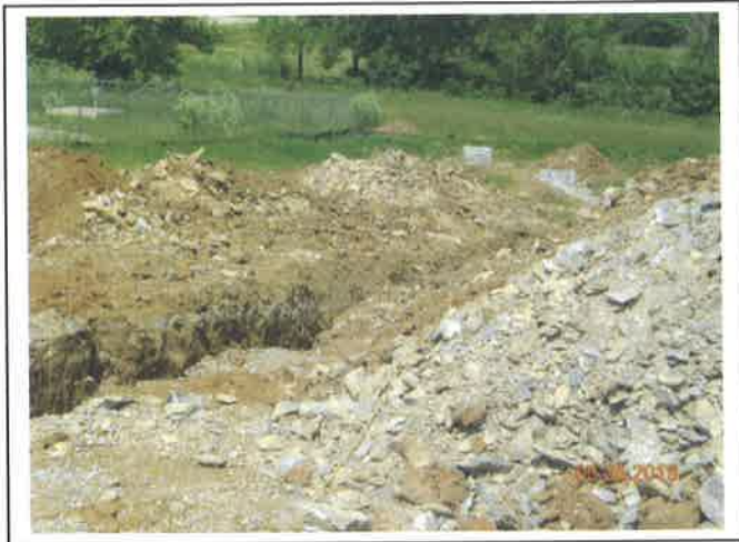
Photo #007 – Rock spoils encountered during Utility excavation (typical)
