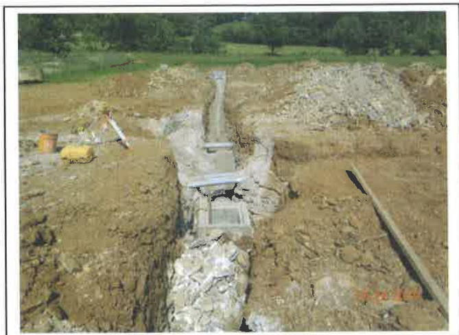
Photo #001 – CB1 to CB2 rock excavation
