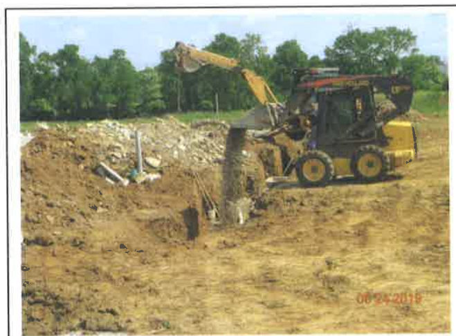
Photo #006 – Backfilling & haunching of Str pipe in progress (typical)
