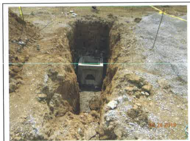
Photo #004 – Catch Basin and work in progress
