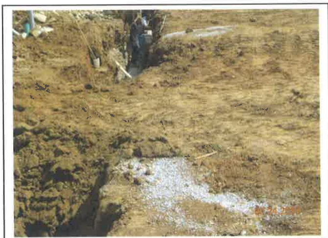
Photo #005 – Str pipe in progress (typical)
