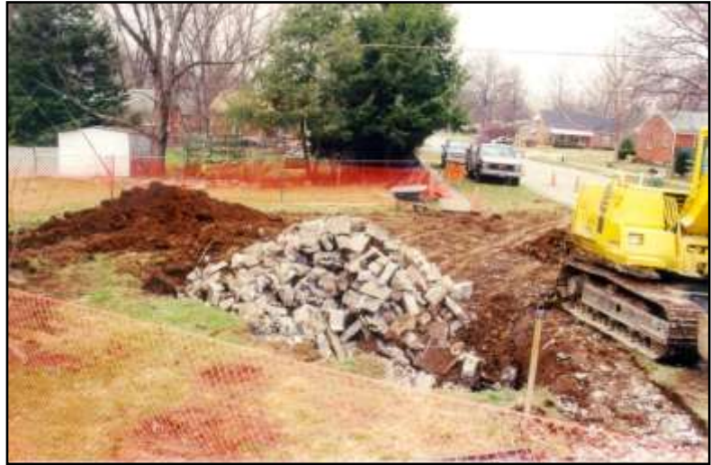
Attempt to fill in a cover-collapse sinkhole.
