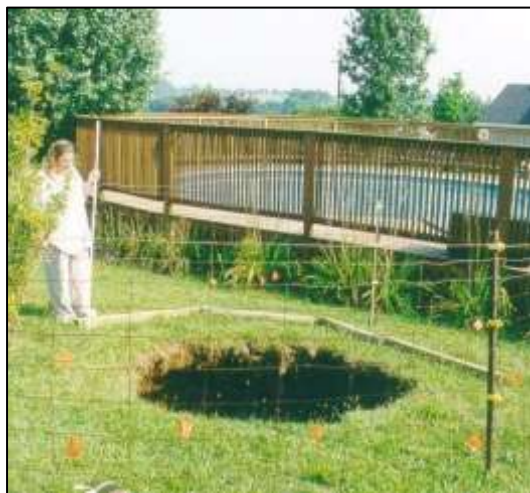
Sinkhole cover collapse in Boyle County. This phenomenon occurs throughout the Inner Bluegrass karst landscape. Source: Kentucky Geological Survey.
