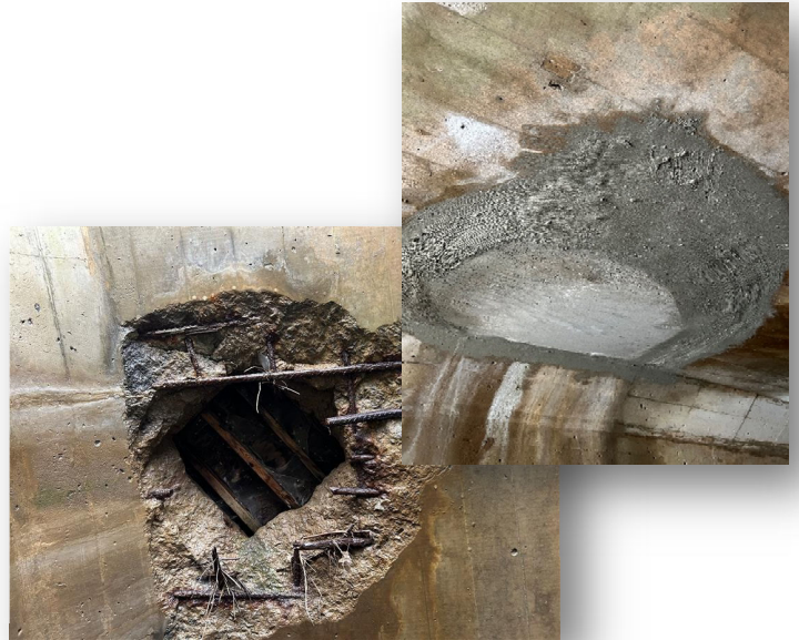
Repaired a Hole In Town Branch Culvert
