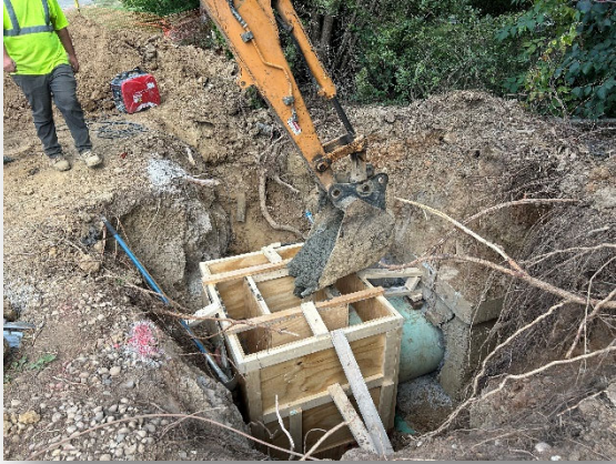
Forming a New Storm Inlet
