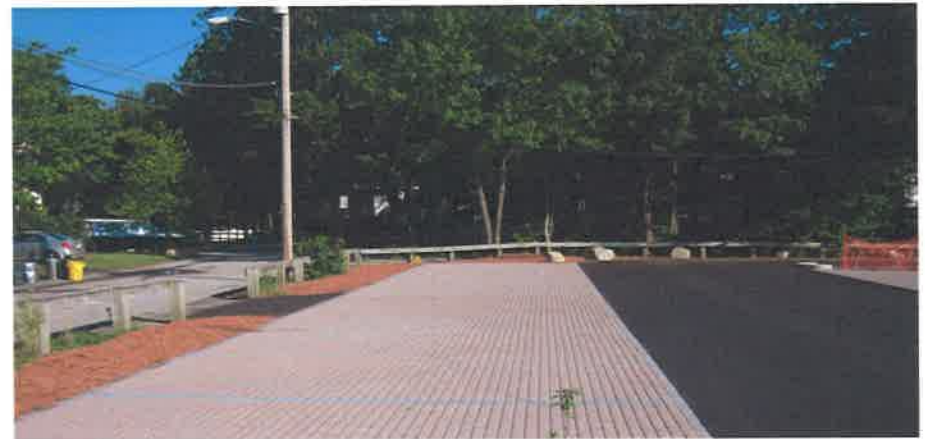
FIGURE #8: examples of green infrastructure options for a parking lot striped at a 90° angle
