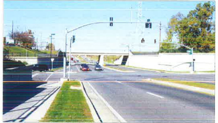
West Reynolds Road Railroad Underpass Reconstruction.
