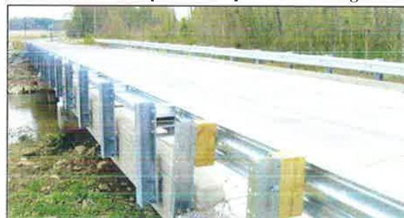
Bean Cemetery Road Bridge Replacement. Madisonville, KY.
