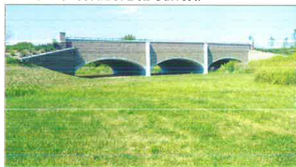
Eastern State Hospital ConSpan Arch Bridge.
