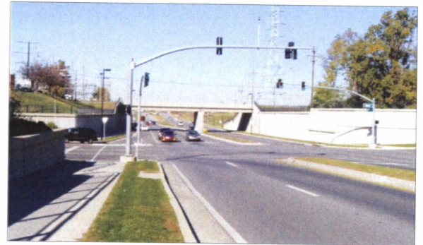
Mall Entrance at West Reynolds Road.
