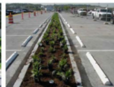
Parking Lot Bioretention
