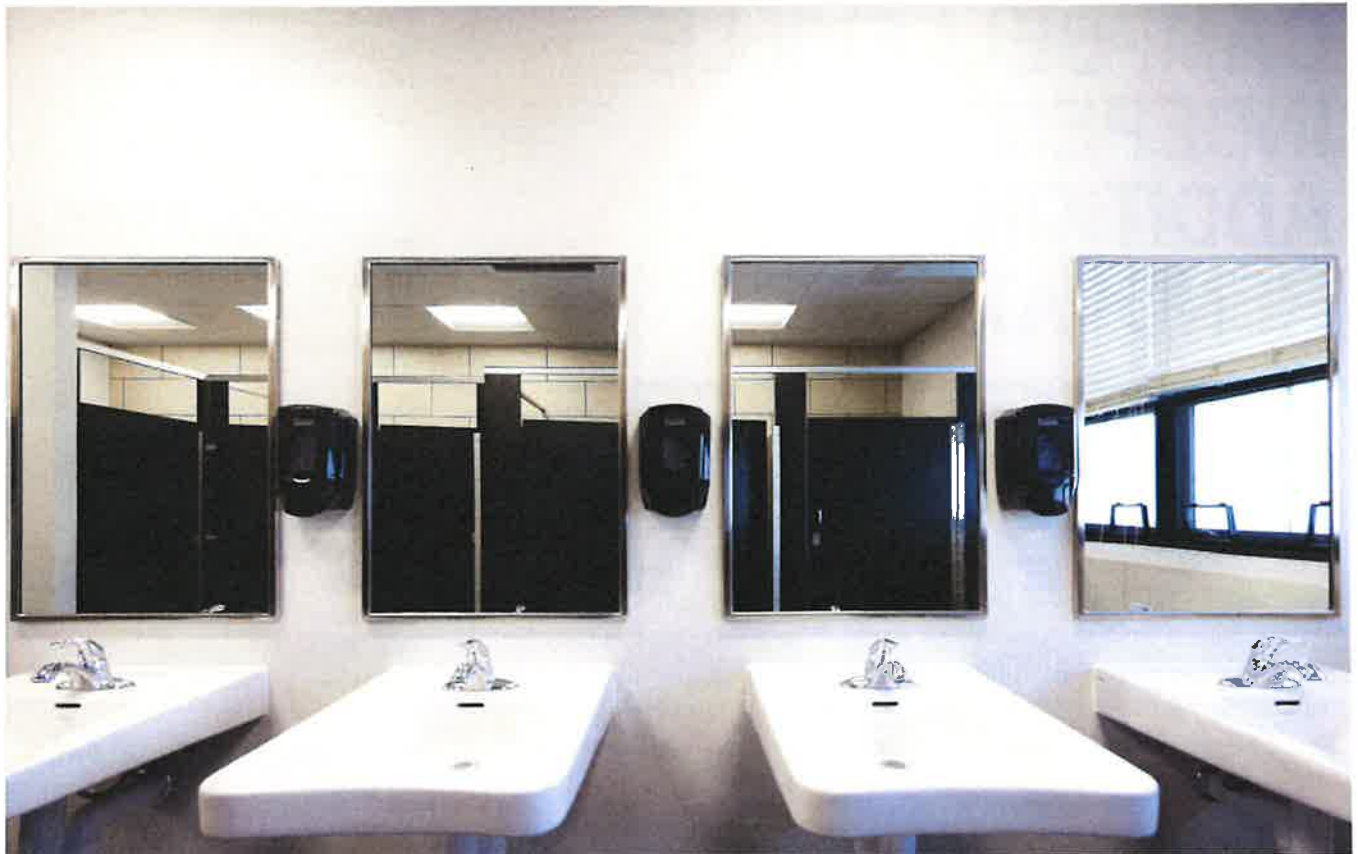
Bottom: First floor restroom plumbing fixtures
