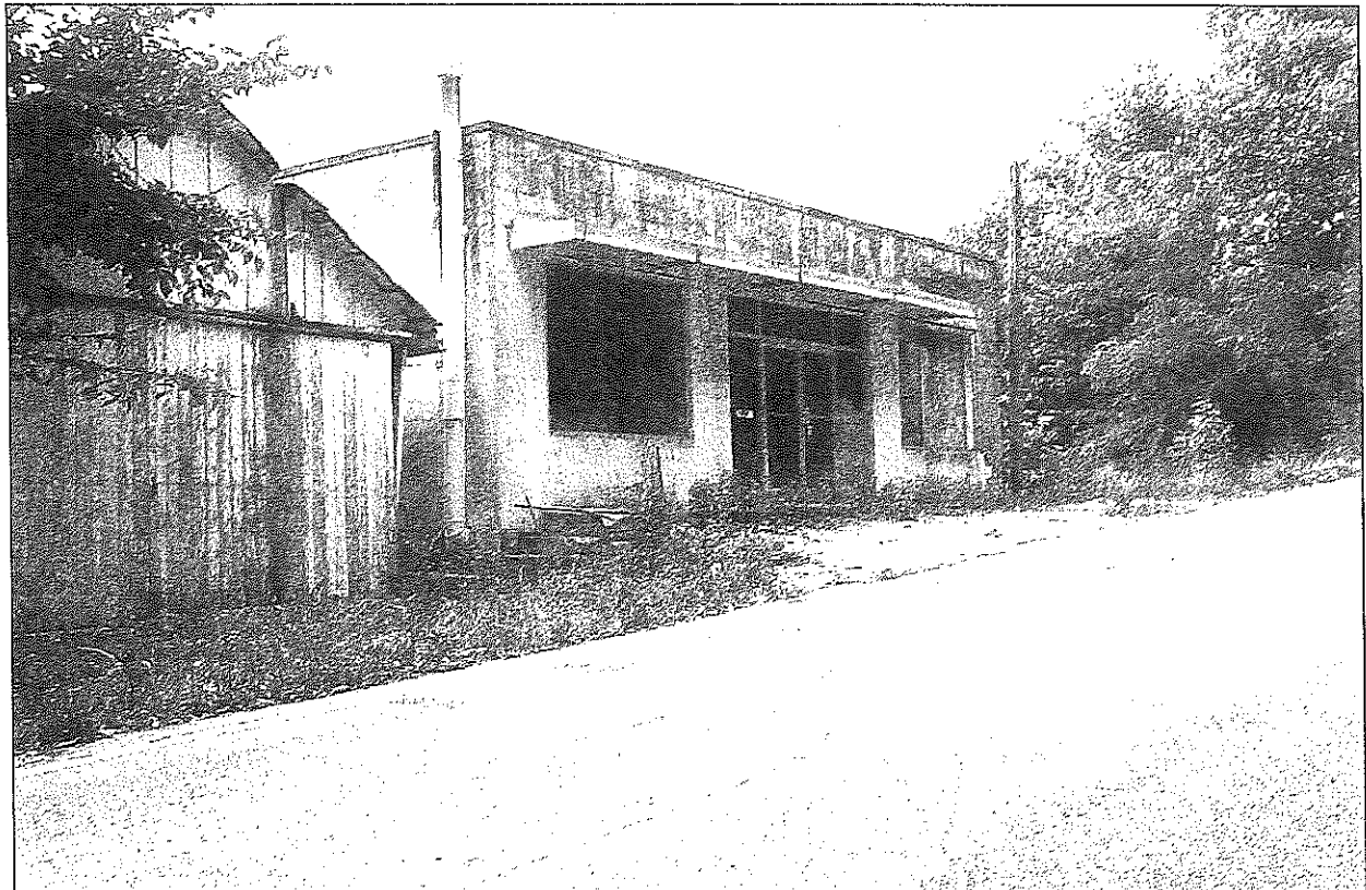
An abandoned store along Old Richmond Rd. near the Kentucky River.
