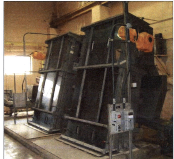
Headworks-Mahr mechanical fine screens.
