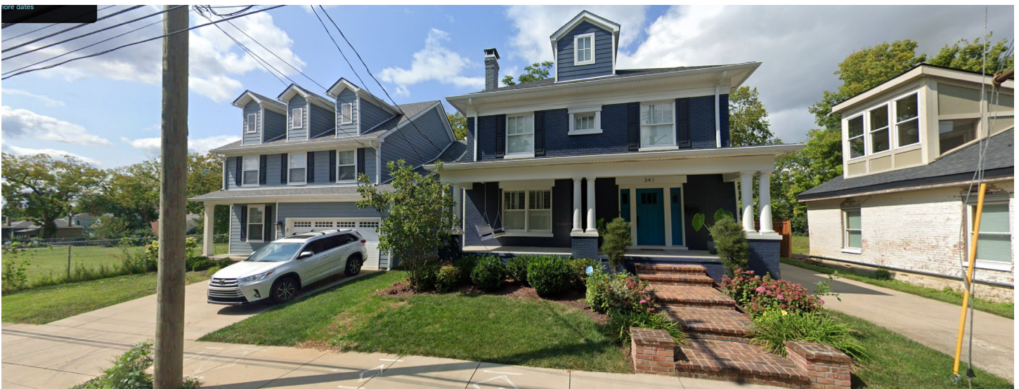
These two houses along North Martin Luther King Boulevard illustrate dramatically different approaches to setbacks, parking access and placement, and overall relationship to the public street. (Courtesy: Google Street View.)
