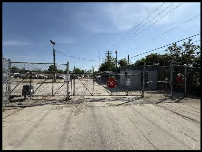
Front Gate with security cameras
