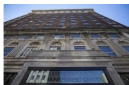
Government Center Building and Garage (153k SF + parking)
