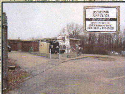
EAST HICKMAN PUMP STATION
