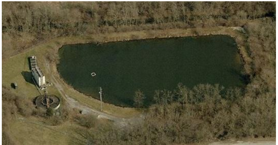
Blue Sky WWTP
