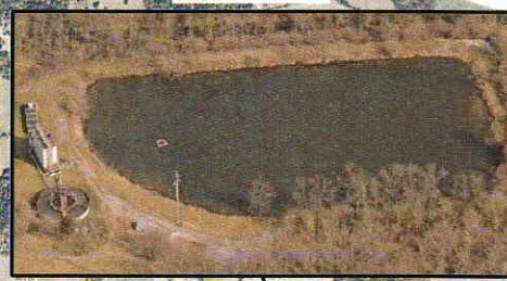
BLUE SKY WWTP
