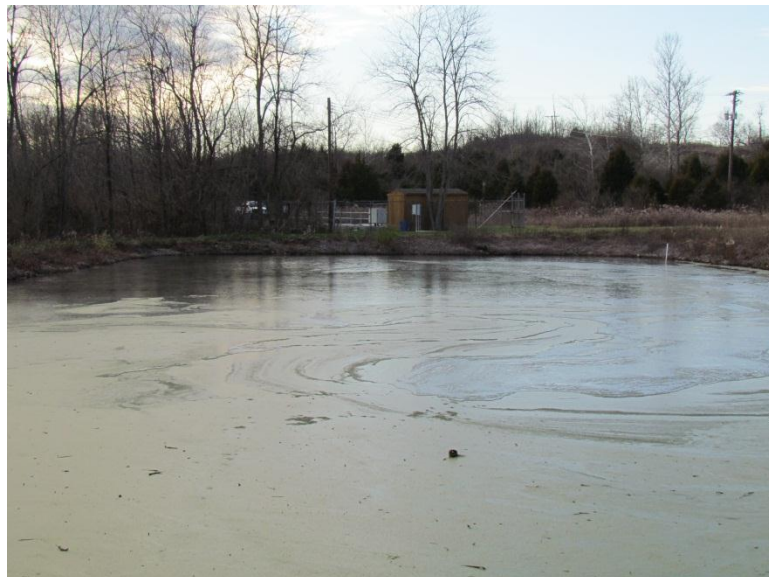
Boonesboro WWTP Lagoon
