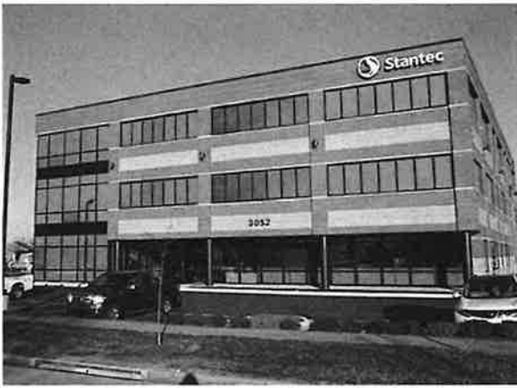
Stantec's Lexington office at 3052 Beaumont Centre Circle
