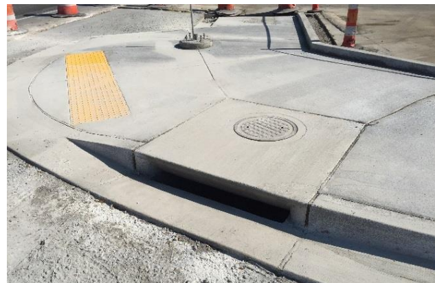
Liberty Road and Winchester Road improved ADA-accessible ramps and storm drainage.
