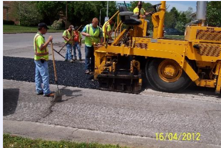
Road Resurfacing Annual maintenance activity
