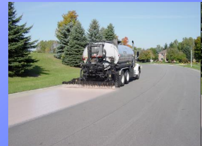
Road Rejuvenation & slurry seal County Maintenance
