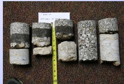
Road Coring Base failure forecasting
