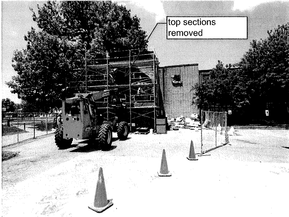
General view during construction. 5/8/15
