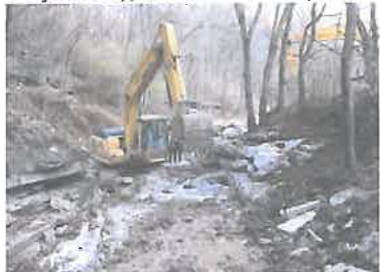
During: construction of rock structures.
