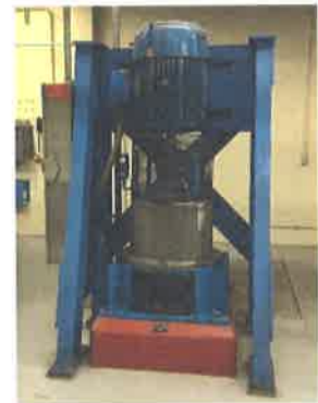
RAS pump motor installation.
