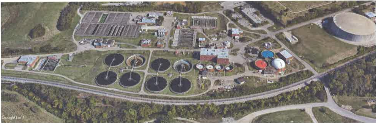
Town Branch Wastewater Treatment Plant.
