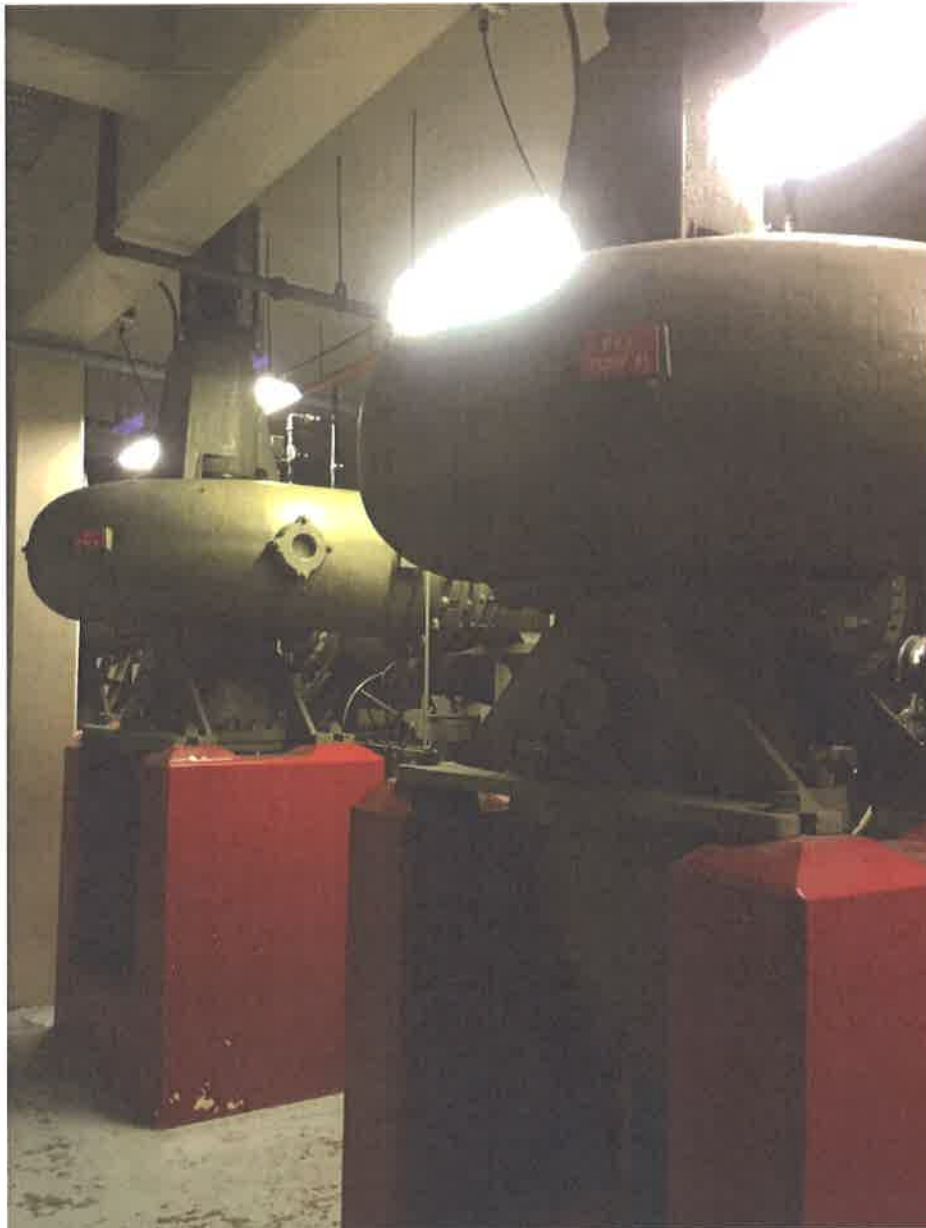
RAS pumps located in lower level.
