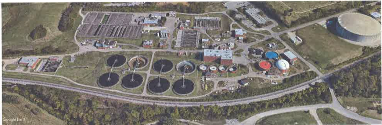
Town Branch Wastewater Treatment Plant.
