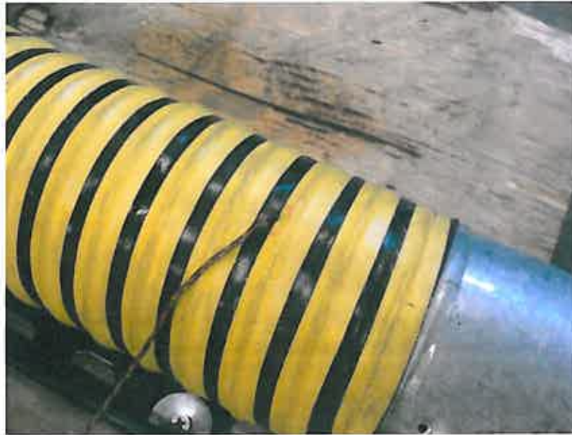
Photo 1 – Attachment of the Hose to the Duct Assembly
