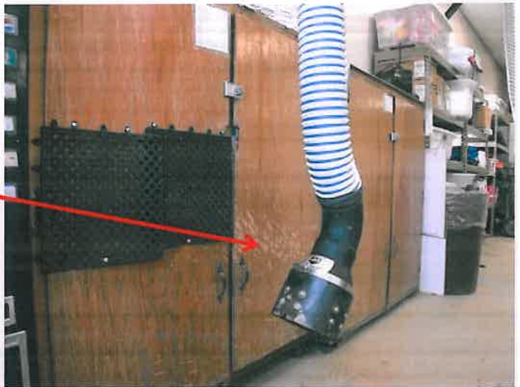
DAMAGE TO CABINETS FROM SWINGING HOSE & NOZZLE
