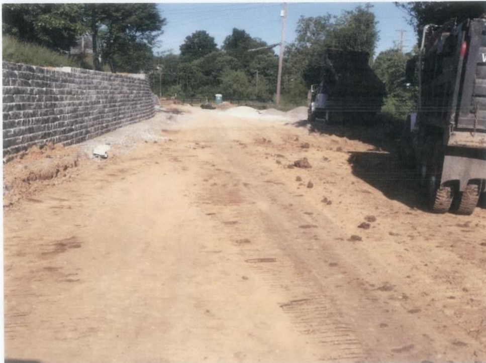
Photo 2: View Of Area Along The Retaining Wall
