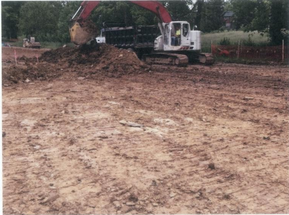
Photo 1: View Of Roadway Being Cut To Grade
