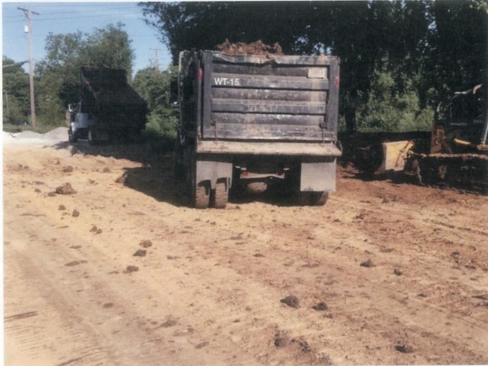
Photo 1: View Of Roadway Being Cut To Grade
