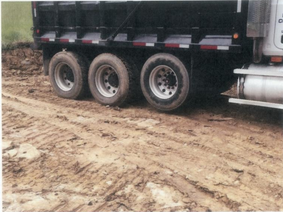
Photo 3: View Of Loaded Truck Performing A Proof Roll To The Sub-Grade
