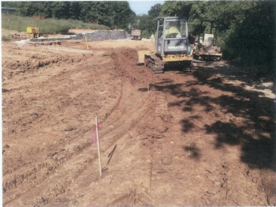
Photo 3: View Of Roadway Being Cut To Grade
