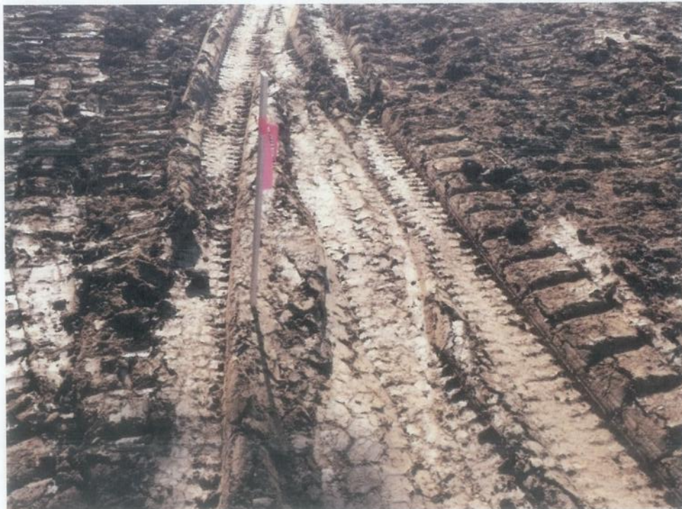
Photo 4: View Of Loaded Truck Performing Proof Roll For The Subgrade
