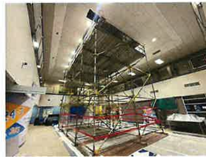
Edgewood: Career Center – Skylight removal & new interior lighting
