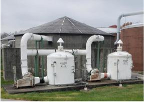
The existing gravity thickener odor control system is activated carbon installed around 1990 with 29,585 pound (max.) dual vessels containing Hetron 922 resin. The condition of the carbon is unknown other than replacement for one vessel reportedly occurred about 18 months ago.
