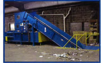
Full Eject Baler Installation at Folding Carton Plant
