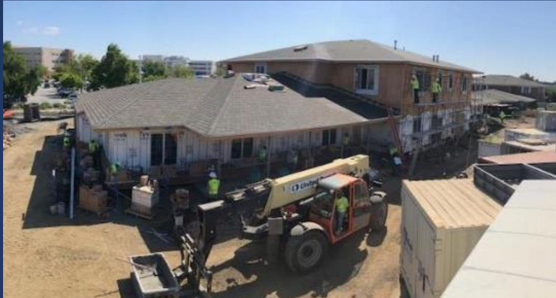
Second Fisher House at Palo Alto CA VAMC currently under construction.
