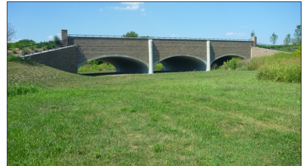
Eastern State Hospital ConSpan Arch Bridge.
