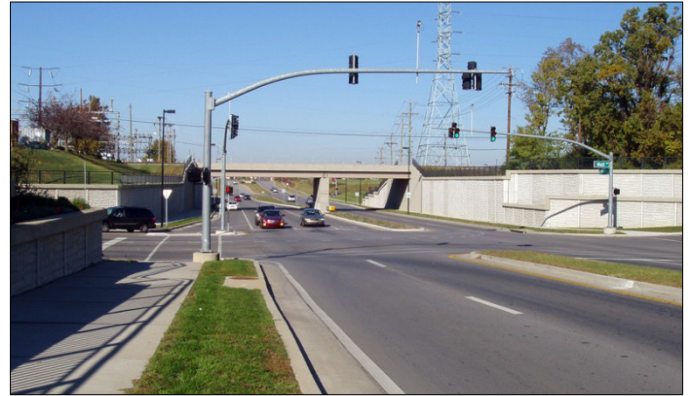
West Reynolds Road Railroad Underpass Reconstruction.
