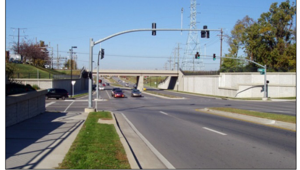
West Reynolds Road Railroad Underpass Reconstruction.
