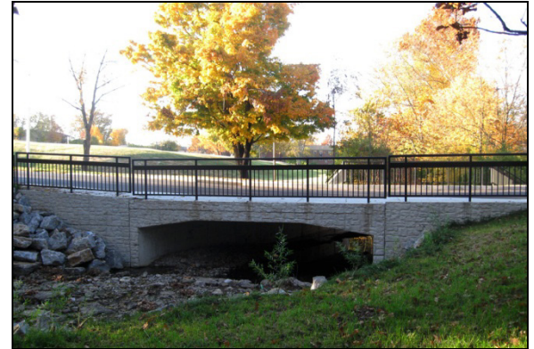
Appomattox Road Culvert Replacement -Double 12-foot x 6-foot R.C. Box Culvert.
