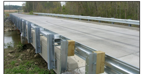
Bean Cemetery Road Bridge Replacement. Madisonville, KY.
