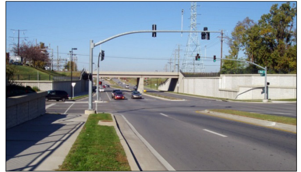
Mall Entrance at West Reynolds Road.
