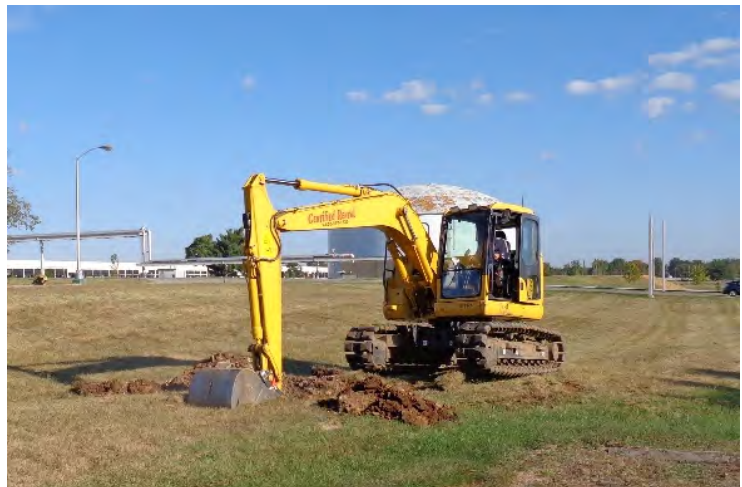
Ridgewater & Stantec advancing a test pit at the Lexmark Rainwater Harvesting System project in Lexington, KY.
