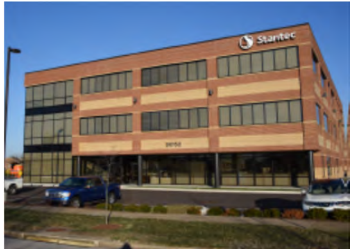
Stantec's Lexington office at 3052 Beaumont Centre Circle
