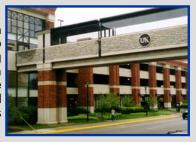
The structures utilized two precast prestressed concrete type III I-beams in the cross-section. This design proved to be a challenge because the beams over Limestone cantilever past the support pier positioned away from the garage. The cantilever was an effective solution that allowed the foundations of the garage and bridge to remain independent. The design required unusual strand configurations to accommodate the stresses produced in the cantilevers.
