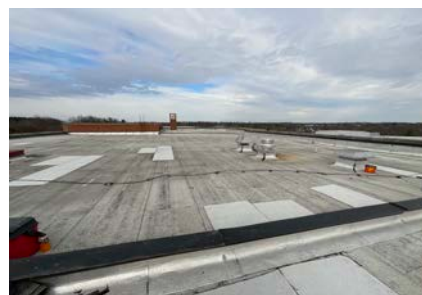
ATB – Roof Repairs
