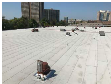
Tech 'B' - Roof
