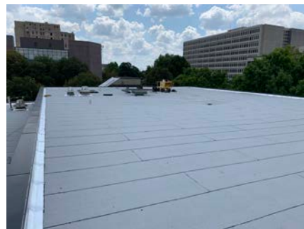
Tech 'B' - Roof
