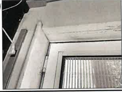
3 INSIDE WINDOW CONSTRUCTION
