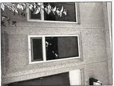
4 OUTSIDE EXIT OF ROOM 121
