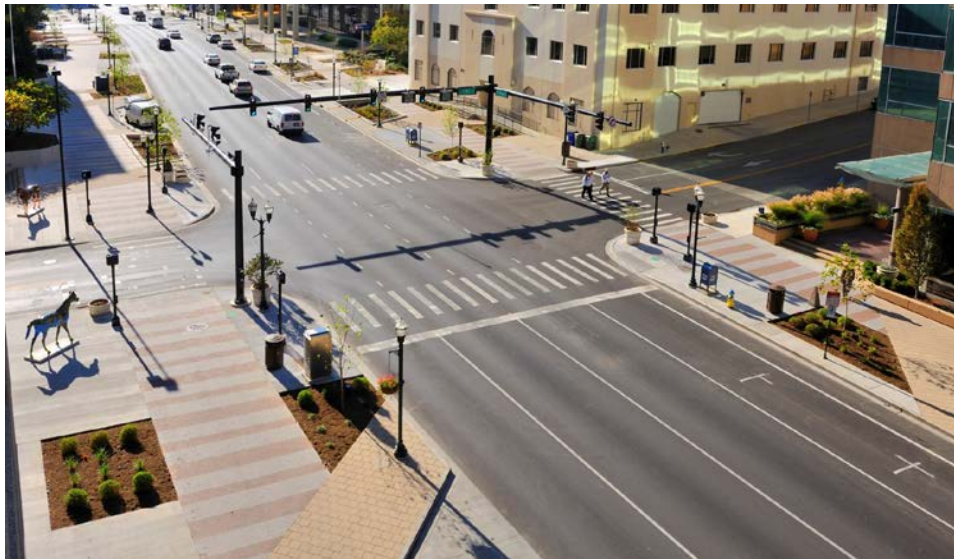
Reconstructed Vine Street and Mill Street intersection.
