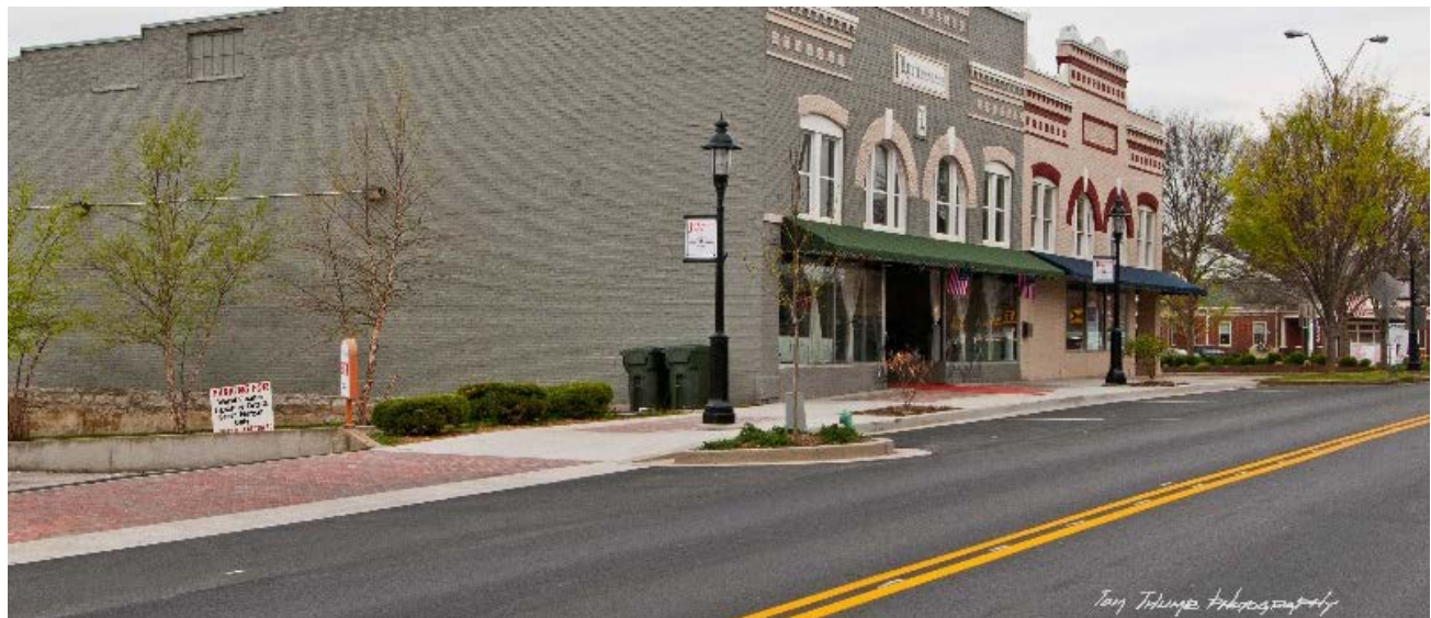
Completed East Main Street.
