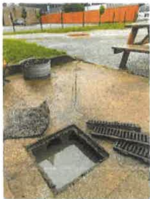
Exterior catch basin – outlet collapsed or nonexistent causes interior flooding
