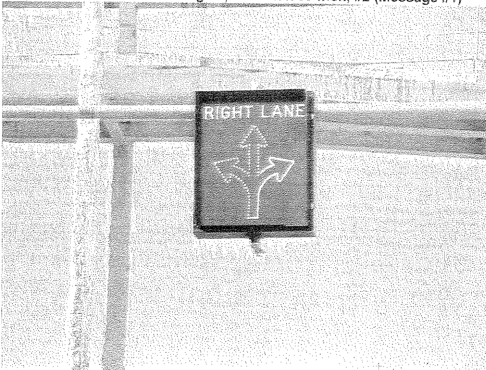
LED Lane Use Control Signal, 30-inch x 36-inch, #2 (Message #1)
