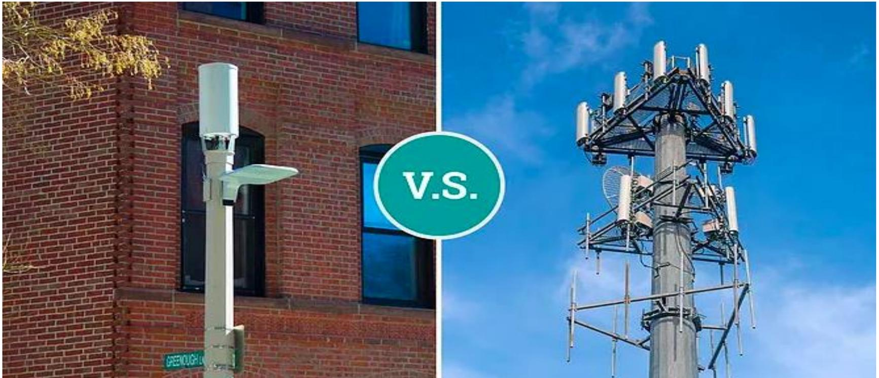
Small cells are portable miniature base stations that require minimal power to operate and can be placed every 250 meters or so throughout cities. To prevent signals from being dropped, carriers could blanket a city with thousands of these stations. Together, they would form a dense network that acts like a relay team, handing off signals like a baton and routing data to users at any location.
