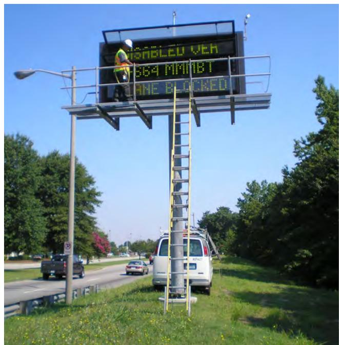
**Installing ITS sign equipment to provide updates to drivers**
