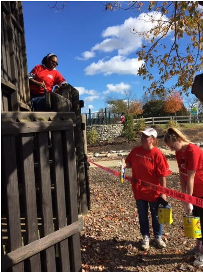
Staining the wooden structure
